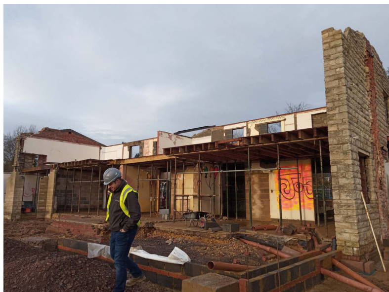
← FIGURE 6: What remained of existing house after demolition
